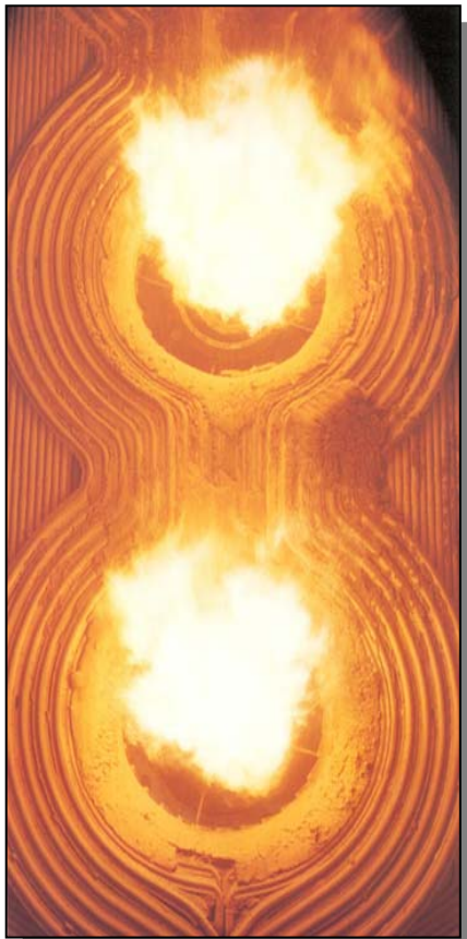
A typical pulverised coal-firing flame
